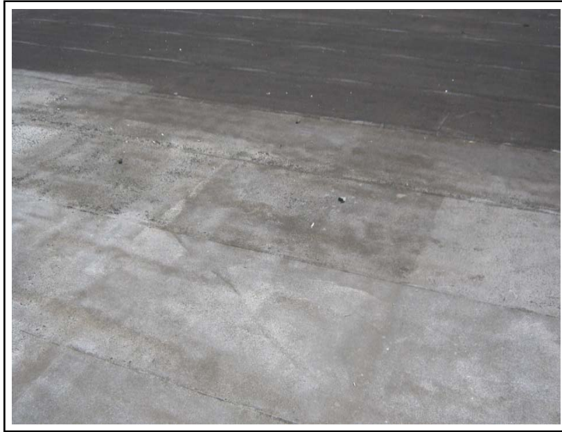
1907-003B-A31: Rolled on Roofing Building B Studio Roof
